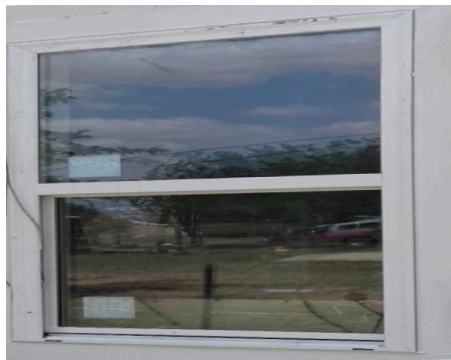
Low E Window installed to replace single pane window.
