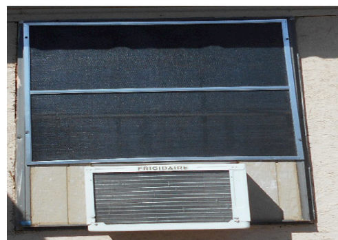
Solar Screen installed.
