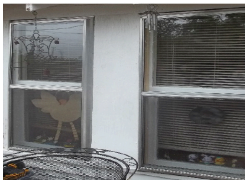
Storm Windows installed over single pane window
